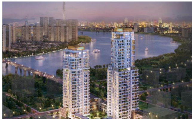
GS Thu Thiem Zeit River (Phase 2) Developer: GS E&C Location: District 2, HCMC
